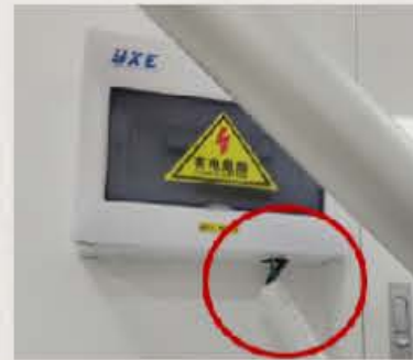
Exposed wiring
