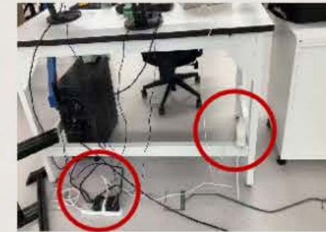
Daisy-chained power strips placed on floors
