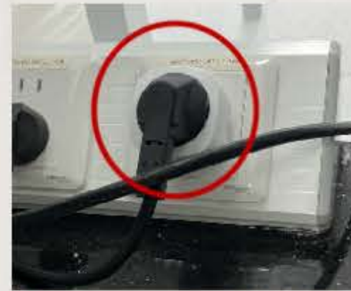
Improper use of 10A-to-16A adapters
